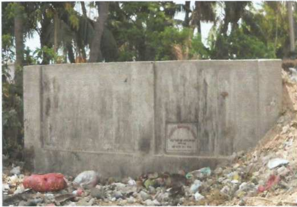
Public Dustbin constructed by M/s Global Coal & Mining Pvt. Ltd., Talcher in village Ghantapada
