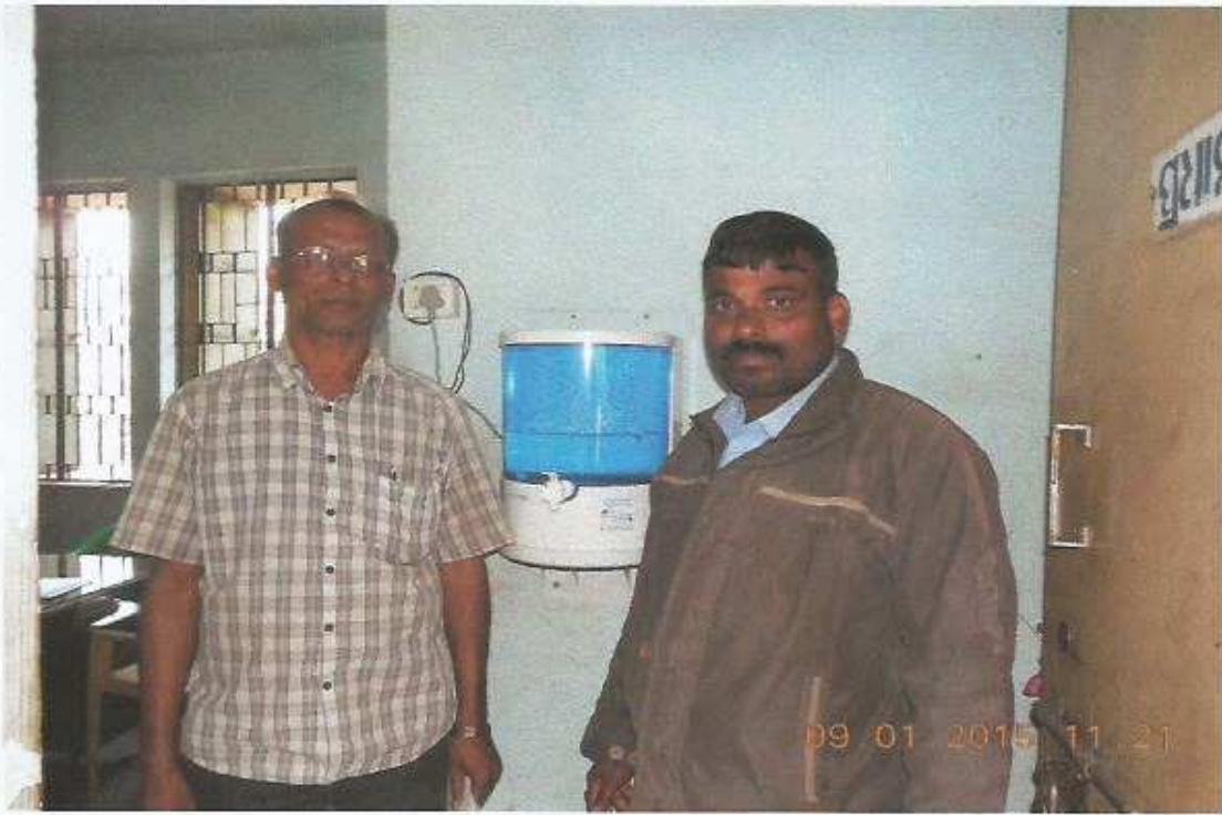
Aquaguard fitted in the school of Central Colony Primary School, Central Colony, Talcher by Global Coal & Mining Pvt. Ltd.
